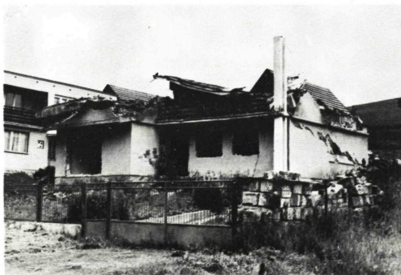
Fig. 22 A disturbed dwelling house situated on the accumulation part of a landslide in the village of Kanská.
