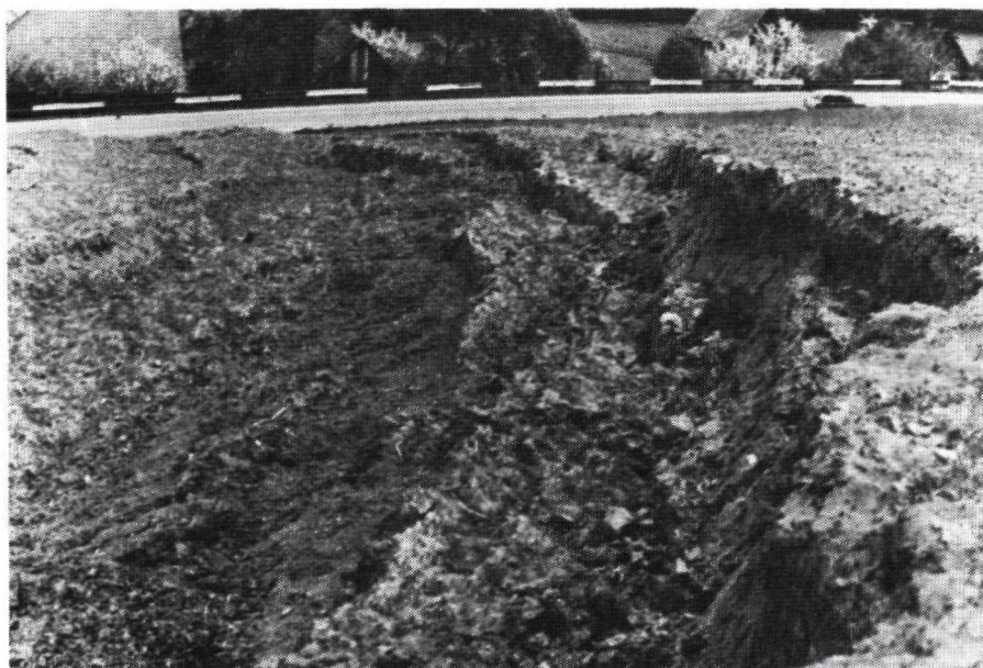
Fig. 5 Rockslide on the southern slope of Mt. Mních triggered by enlarging a railway station at Ružomberok in 1949
