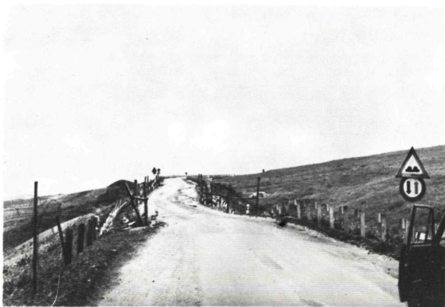
Fig. 7 A road near the village of Věterná Poruba disturbed by an active landslide
