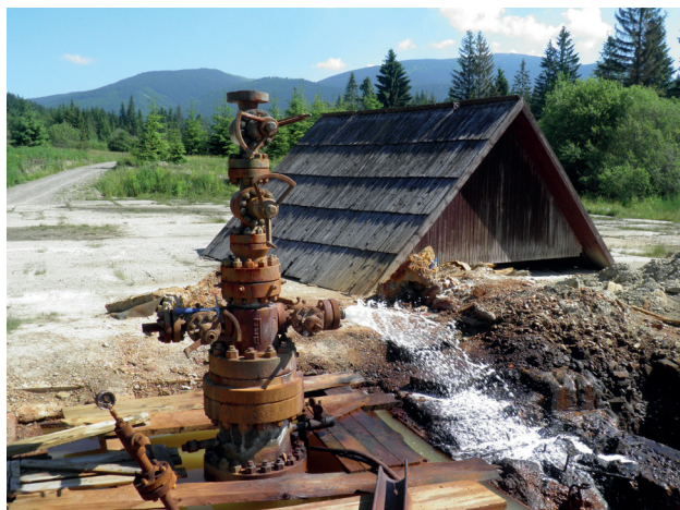
Fig. 1.2 Wellhead of borehole FPJ-1 Oravská Polhora – Slaná voda (Photo: Teťák, 2012, in Teťák et al., 2016)
