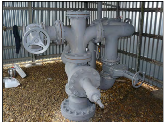
Fig. 4.8 Reinjection well in Podhájska GRP-1 (Photo: D. Marcin, 2012)
