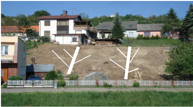
Fig. 1.5 Configuration of stabilization-drainage ribs at the site Krupina
