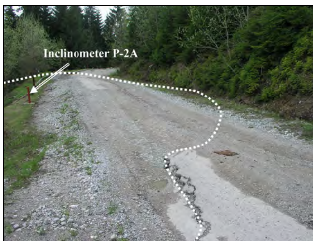
Fig. 8.13 Main scarp area of the active landslide in the body of the forest road with inclinometer P-2A
