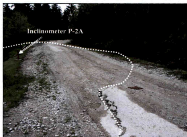
Fig. 8.13 Main scarp area of the active landslide in the body of the forest road with inclinometer P-2A
