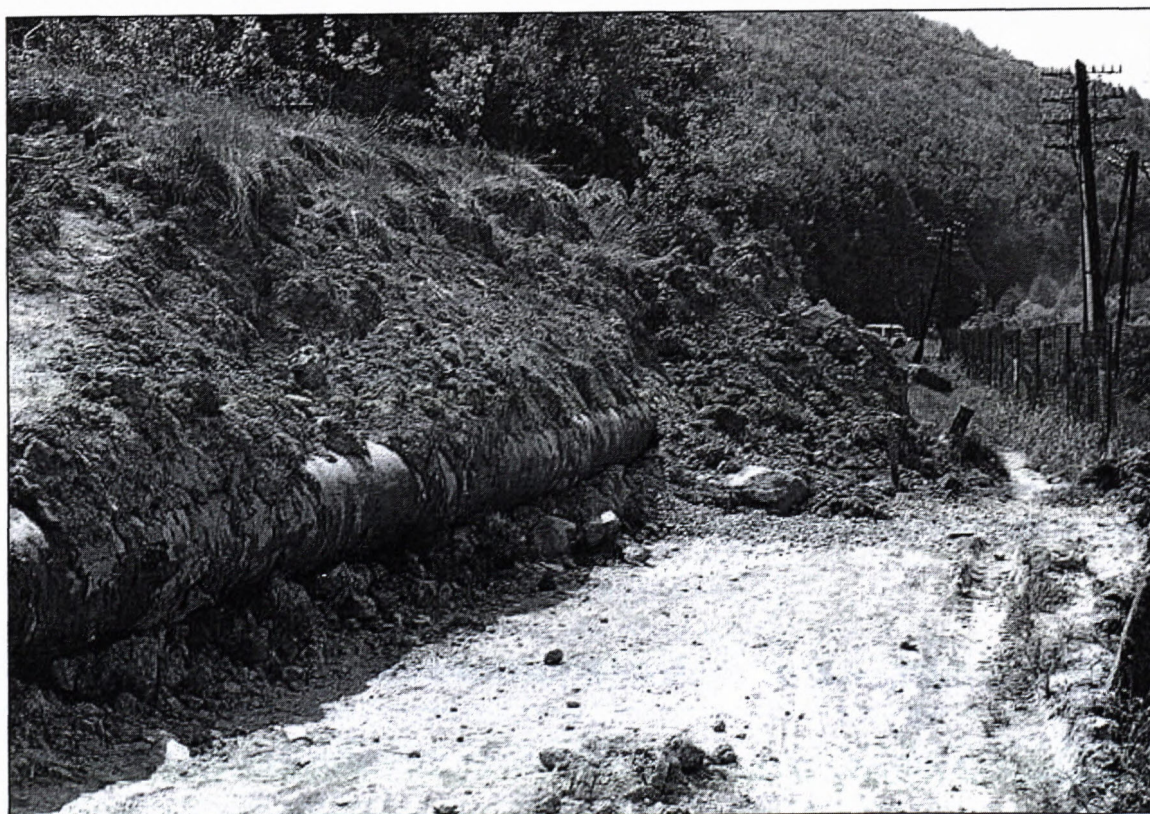
Fig. 6. Water-pipe in accumulation of landslide near Hrinova dam (April 2000).
