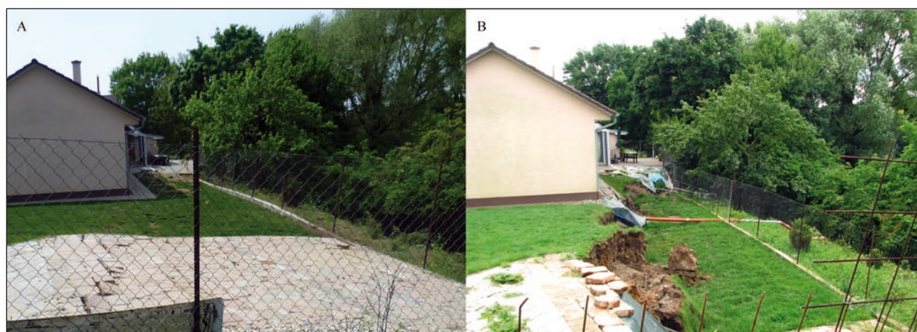
Fig. 10. Family double-house endangered by the landslide in Vinohrady nad Váhom – part Kamenica. A – recorded on 28. April 2011 (Photo M. Bednarik); B – recorded after Declaration of Emergency Situation, 22. June 2011 (Photo P. Ondrejka).
