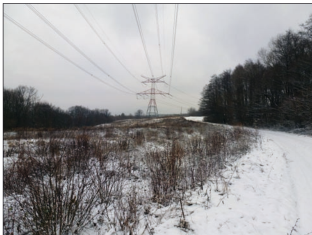
Fig. 3. Jeopardized VHV mast (400 kV) erected in 2011, located in the transportation part of the active landslide. Photo L. Petro, December 2011.
