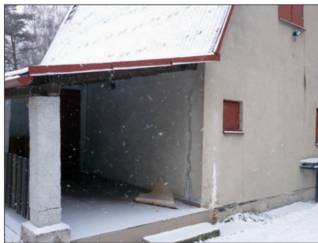
Fig. 4. Static breach of the cottage in the forest-park near Ruská Nová Ves. Photo L. Petro, December 2011.
