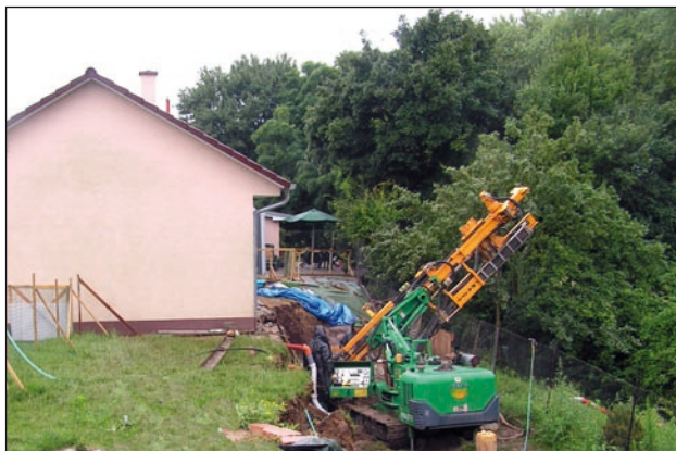
Fig. 12. Remedial works aiming on the rescue of the family double-house No. 711 a 712 (construction of the anchored micro-pile wall). Photo I. Dananaj, June 2011.
