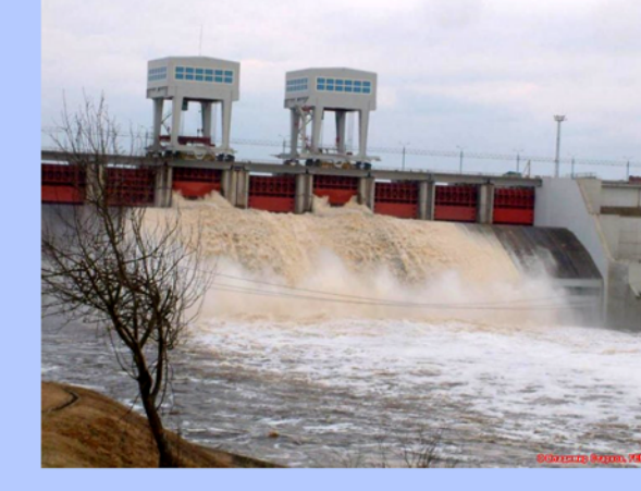
Hydro Power Plant, Latvia
